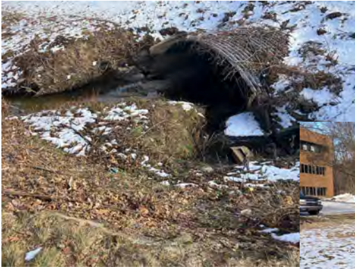
Soil deposition -> loss of capacity Erosion
