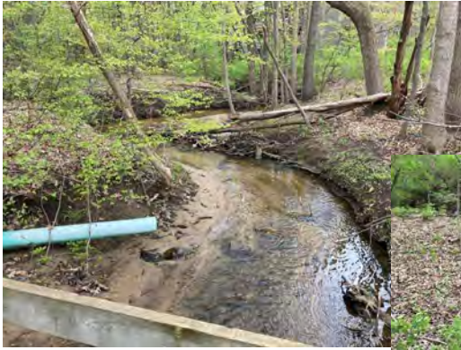
Undermining drain pipes Soil deposition , point bars
